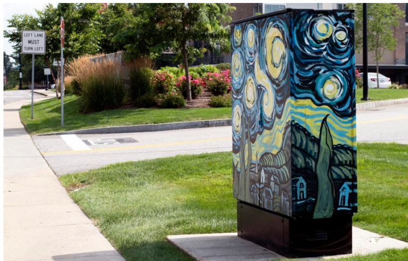
A rendition of Van Gogh's "Starry Night" is painted on an electrical box near the Solaris Renewables office in Burlington, MA.
